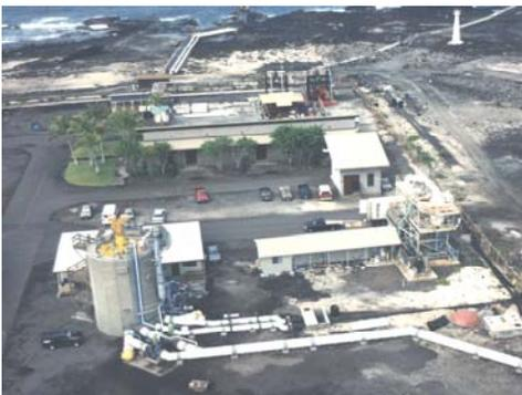
Aerial view of the largest experimental OTEC plant to date. It was built and operated at Keahole Point, Big Island of Hawaii, through the mid-1990s.
